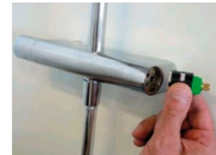
4. Insert the new cartridge
